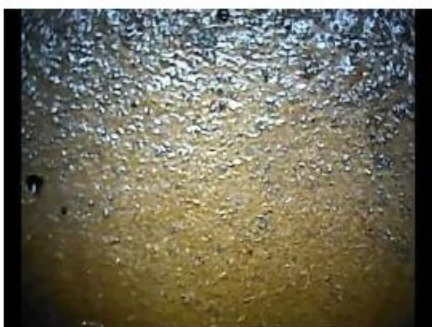
3) End Point gully4
