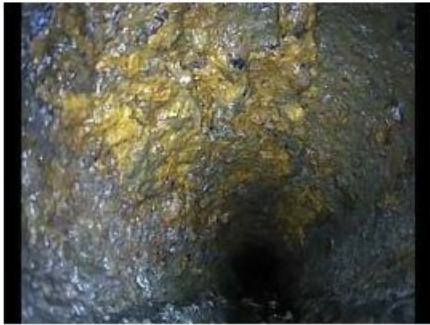
1) Start Point MH3
