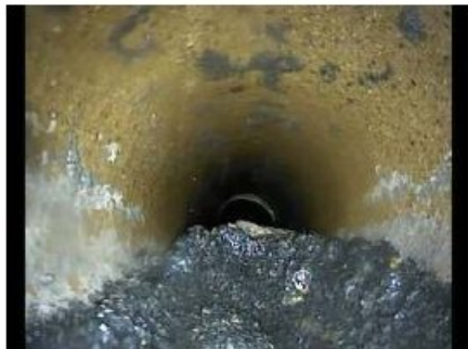
1) Start Point MH3
