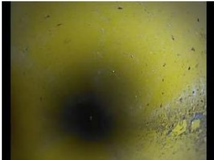
1) Start Point MH1
