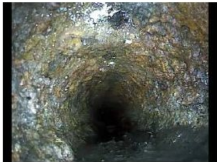
1) Start Point MH3
