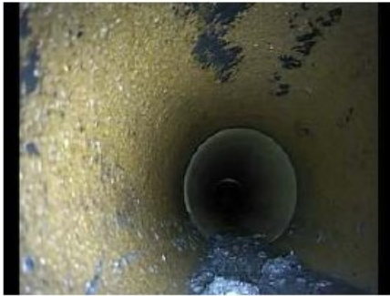
1) Start Point MH4
