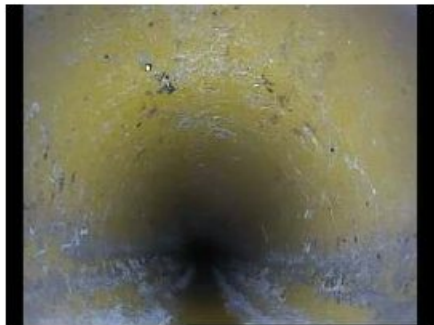
1) Start Point MH1
