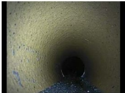
1) Start Point MH4
