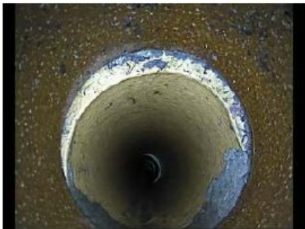
1) Start Point MH4
