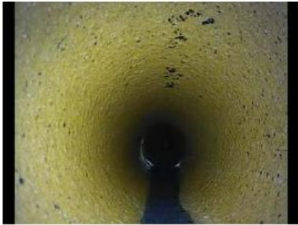
1) Start Point MH3
