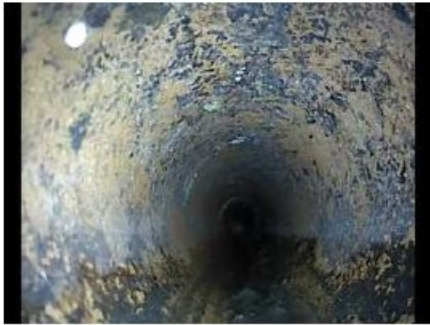
1) Start Point MH4
